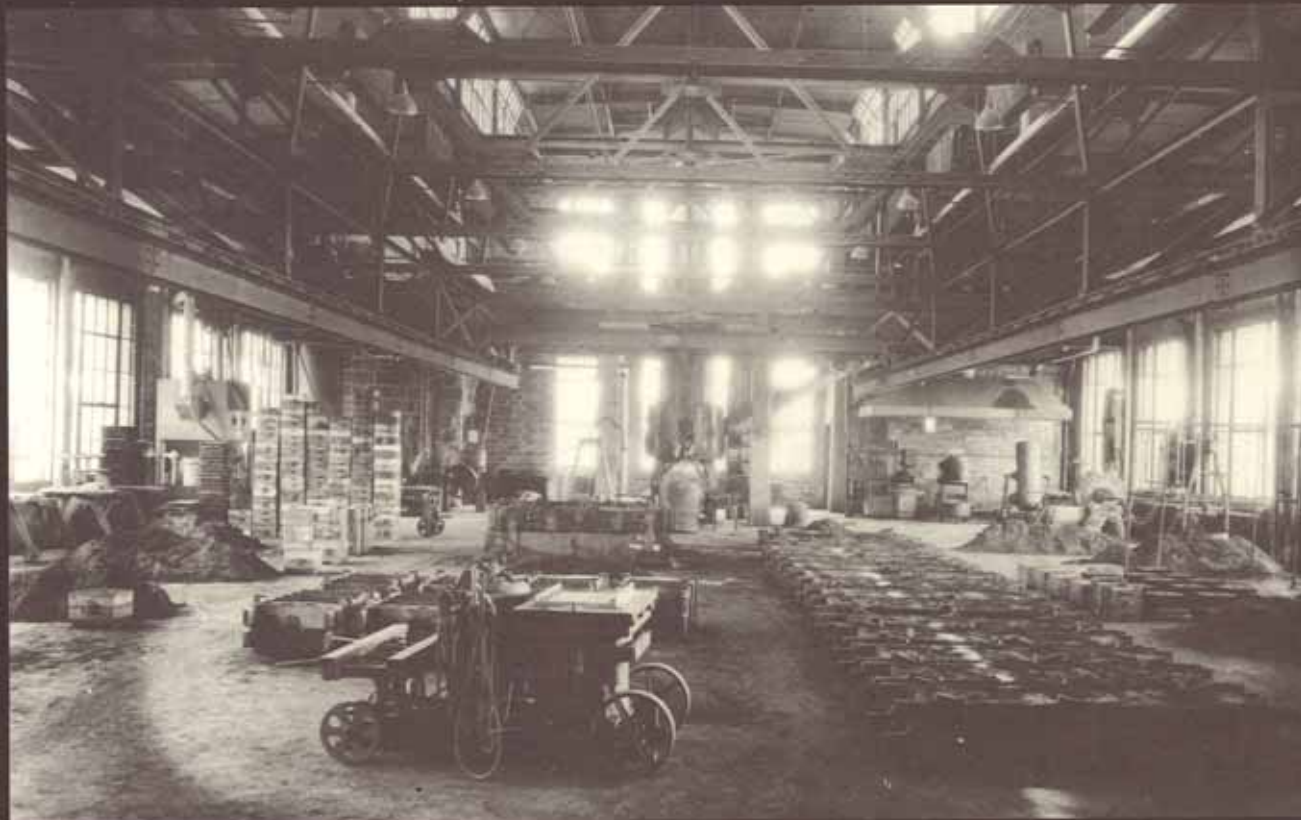
Boston was given the task of redesigning the foundry of the Engineering Laboratory. These photos (taken the spring of 1924) show the foundry as laid out by Boston assisted by H.L. Campbell and John Grennan.
